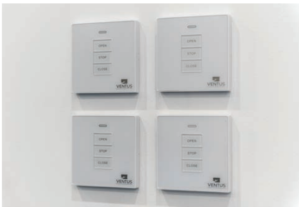
Four panel controls manage each window section which have up to eight chainwinders each
